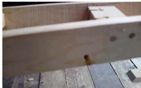
*Figure 9. Dowels and lashings to secure each deck beam*
